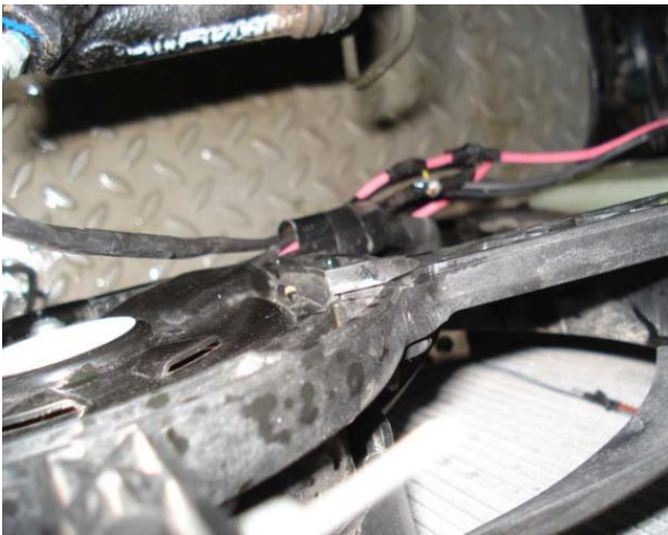
Figure 6: The voltage of fan on the vehicle
